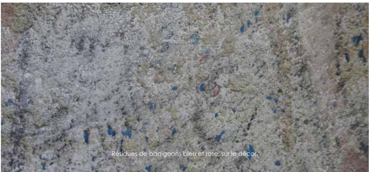
Efflorescences salines.
